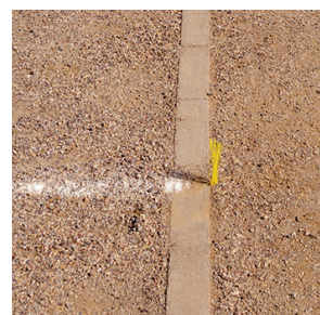
Use of landscape blocks for shooting lines. Paseo Vista Recreation Area Chandler, Ariz.
